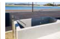
The icing bath The facility is used for cooling down.
